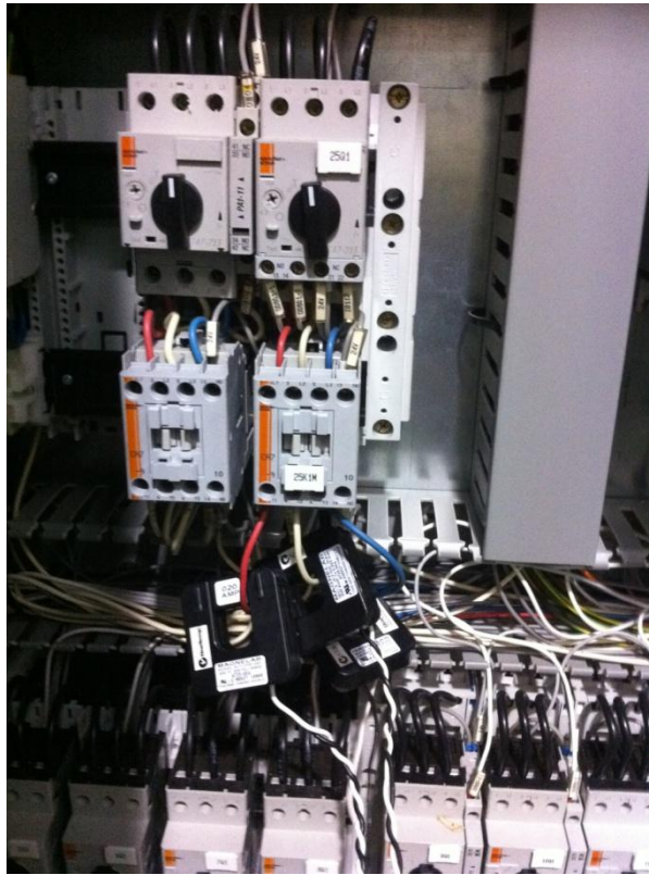
Figure 2.6: Current clamps connected to brine distribution pump power supply
