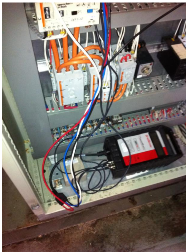
Figure 2.5: Power logger connected to refrigeration plant power supply
