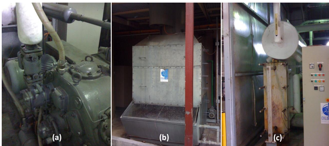
Figure 2.3: Key refrigeration plant components: (a) Compressor, (b) Condenser, and (c) Evaporator
