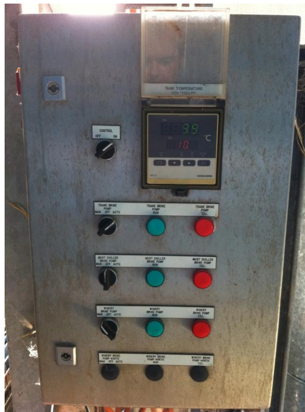
Figure 3.4: Winery control panel for cooling/brine reticulation system
