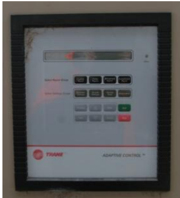
Figure 3.3: Factory-fitted packaged chiller control pad and display
