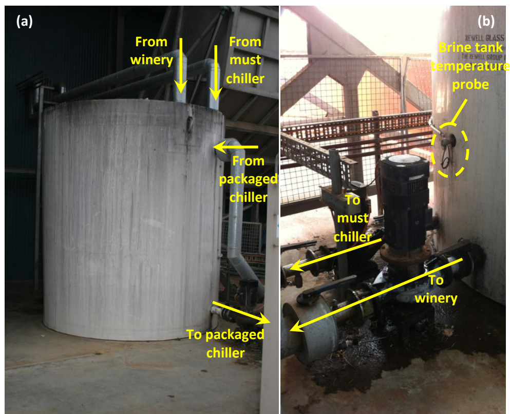
Figure 3.2: (a) Brine tank, (b) Close up on opposite side of brine tank showing brine pumps servicing the must chiller and the winery
