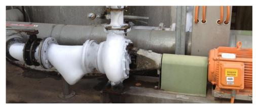
Figure 2. Ice forming on a short section of the system that is not insulated
