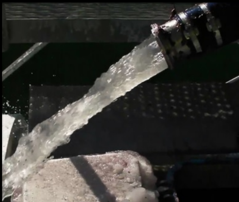
Push water following an ice pig
