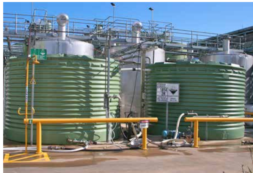
Caustic solution storage tanks
