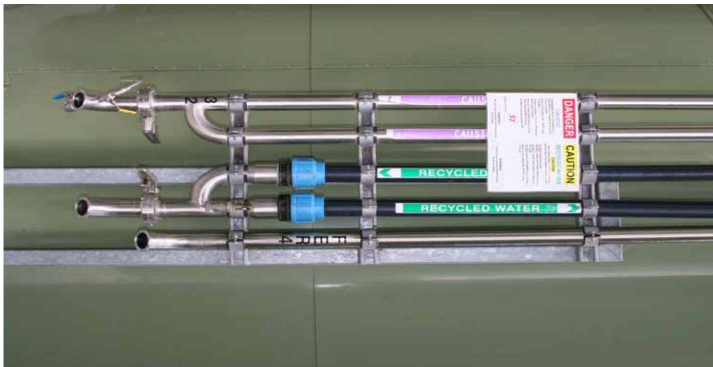
Fixed Caustic and Cleaning Water lines for recycling
