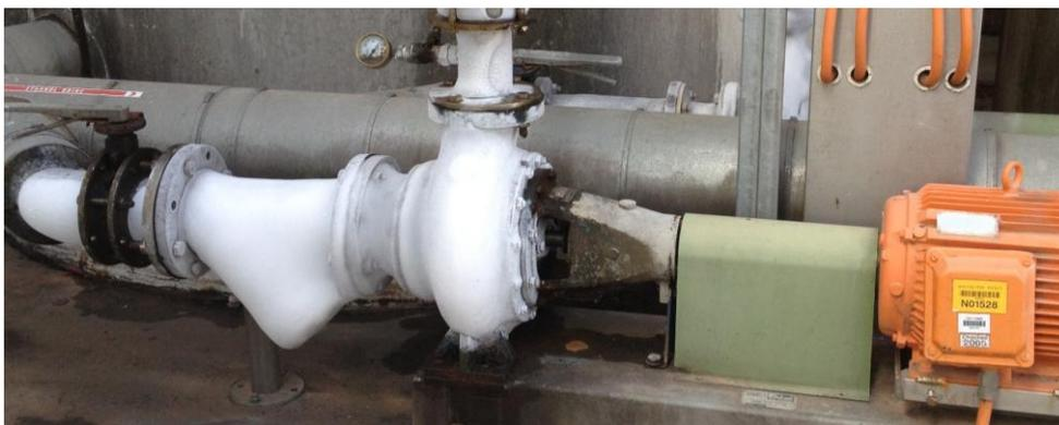
*Figure 2. Ice forming on a short section of the system that is not insulated*
