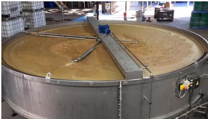
Continuous separation basin with rotating suction heads to remove floats – new installation (2017)
