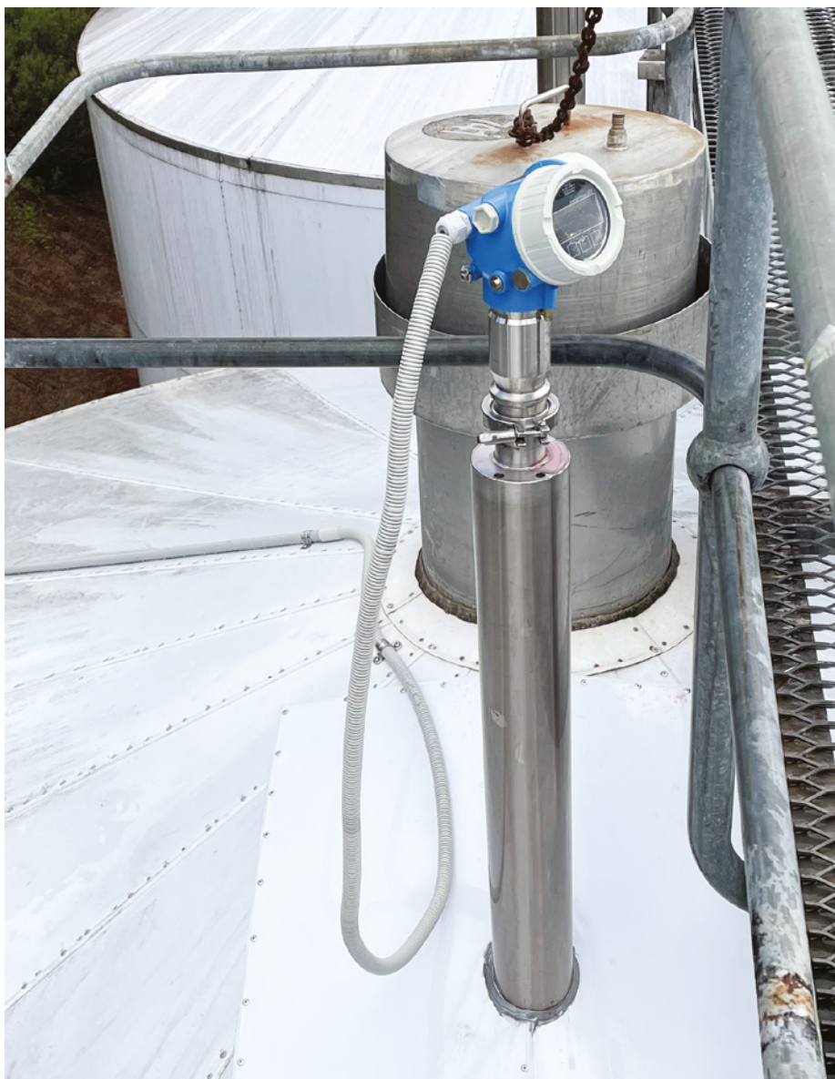
Figure 5. Radar positioned on an extension tube to allow level measurement up to tank brim without obstructing the tank lid
