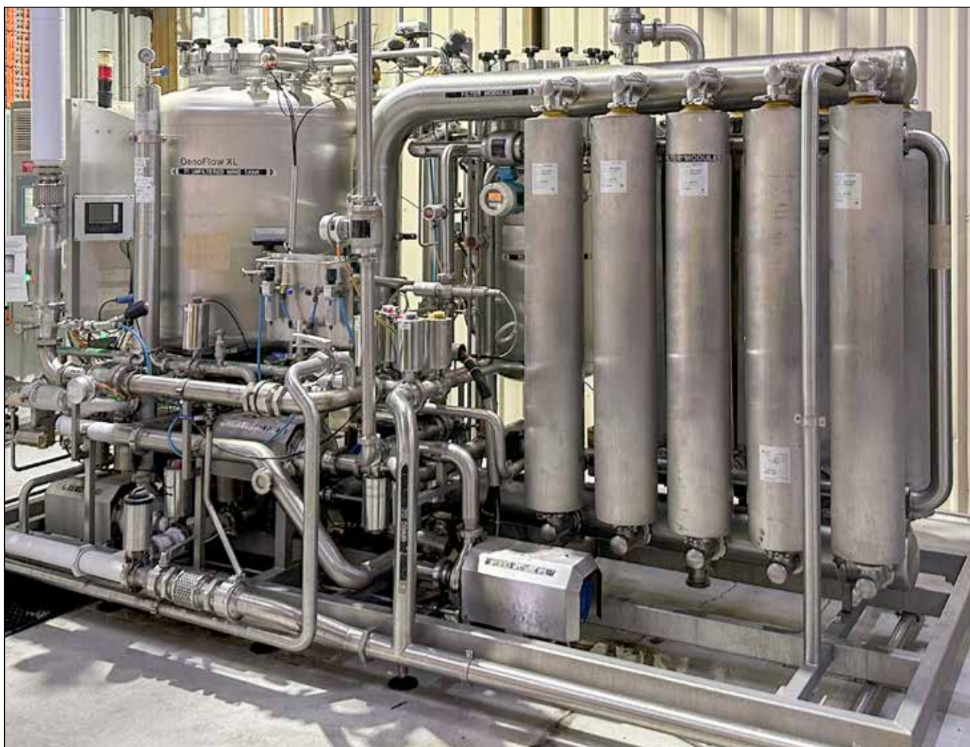
Figure 4. Cross-flow filter for isobaric sparkling wine clarification at a winery
