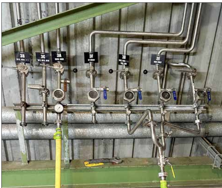
Figure 5. Headspace key station at another winery
